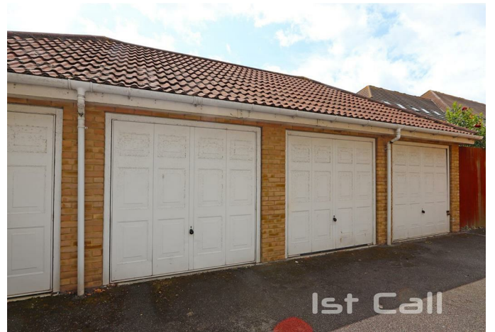
Off Street Parking & Garage
